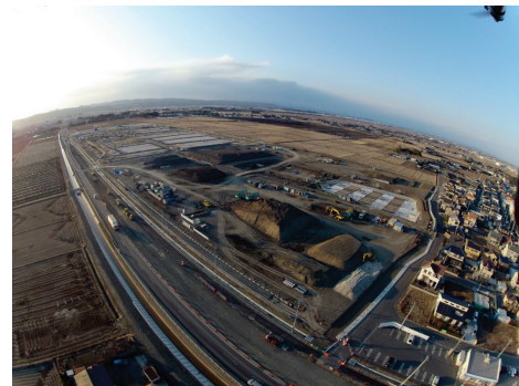
Fig. 6 The relocation project taken by the UAV
