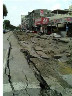
Figure 2. A road section in the explosion area
